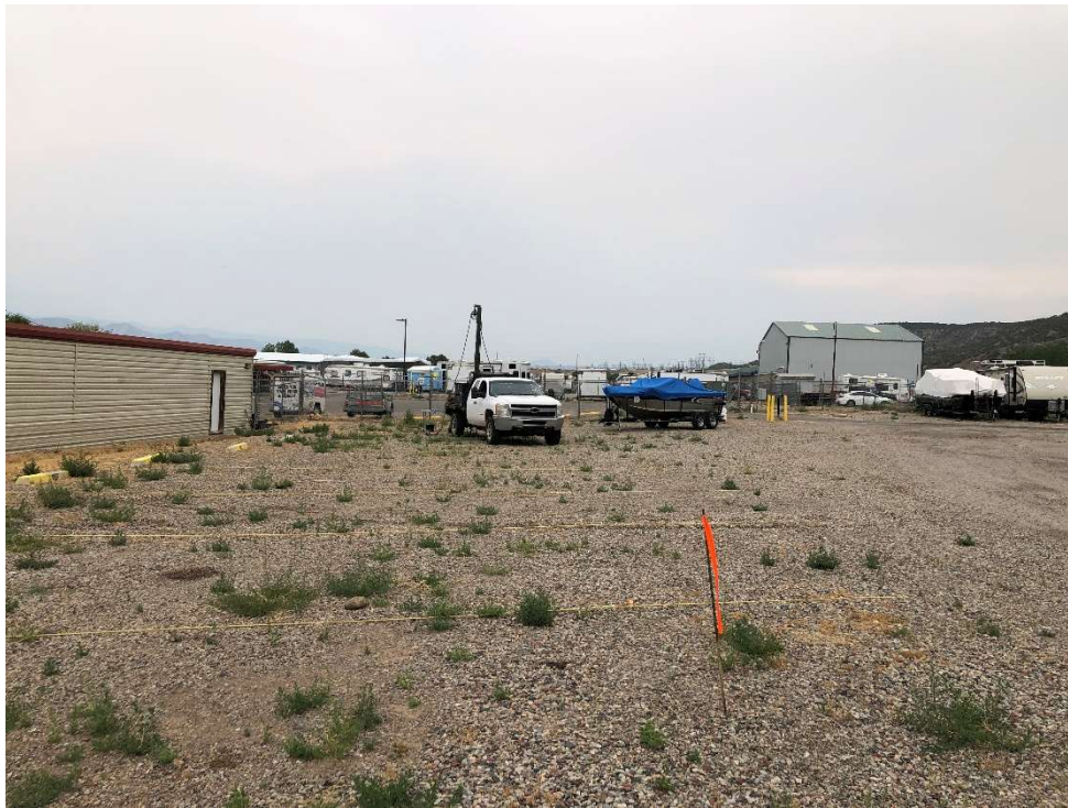
Figure 2 –Drilling Boring B-4, Looking East
